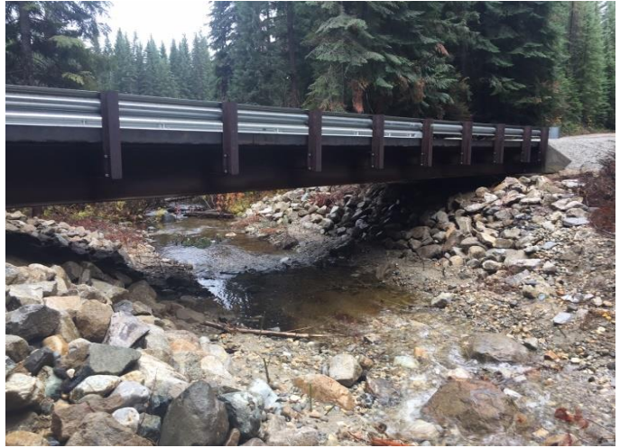
Minnow Creek Bridge
